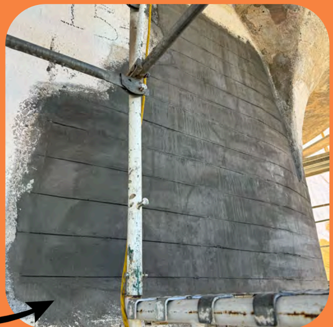
Upper Left: Current KML covered in scaffolding while under construction Upper Right: Project signage at the front entrance of KML. Lower Left: Deteriorated concrete removed exposing original reinforcement rebar. Lower Right: Newly patched concrete spall.
